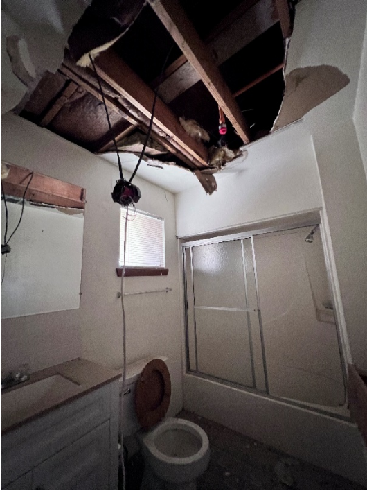
2. Exposed wiring in one of the common areas
