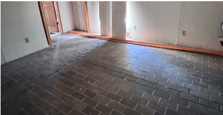
4. Inside of a unit showing the floor buckling and cracking
