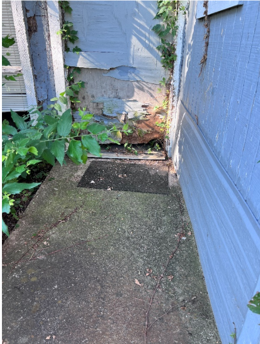
2) Holes in the doorway of units
