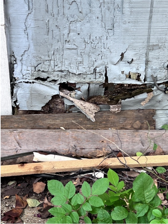
2) Holes in the doorway of units
