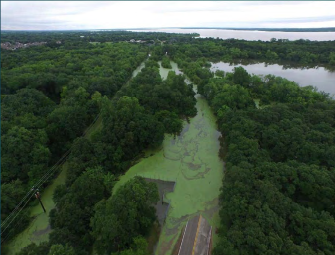
S Shady Shores Rd at LCMUA Lift Station #7 Looking North towards Town Hall
