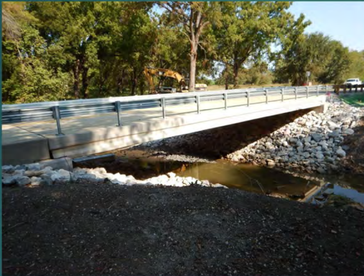
Sample 60-foot Long Single Span Bridge in Collin County
