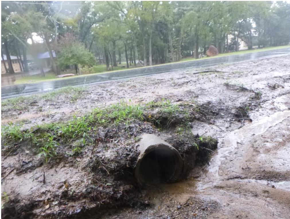
Photo 3: View, facing west, of the culvert that runs under Hidden Valley Road.
