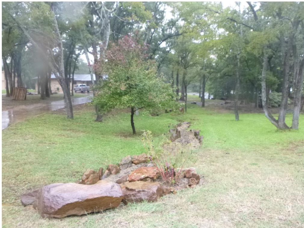
Photo 4: View, facing west, of the man-made drainage channel located on the western side of Hidden Valley Road.
