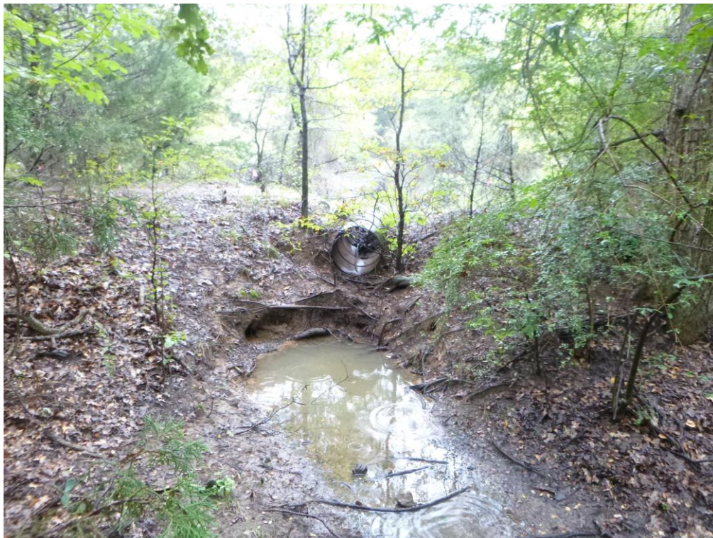
Photo 2: View, facing east, of the culvert and drainage swale located at T2P2.
