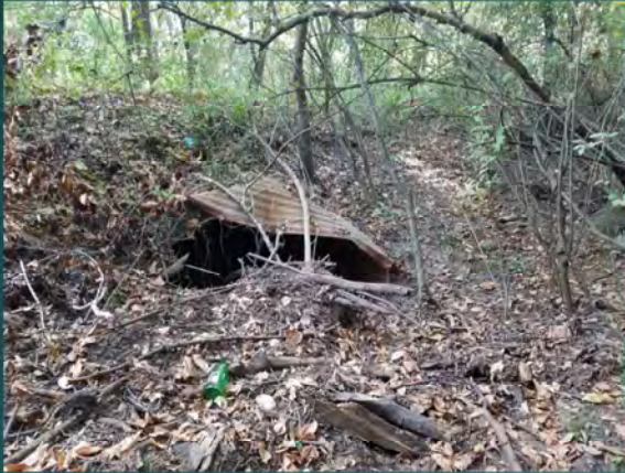
Upstream (south) side
