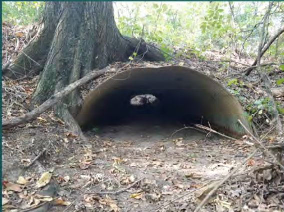
Downstream (north) side
